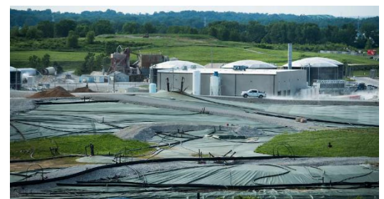
(iv) EPA Orders Cleanup at St. Louis Nuclear Waste Site - Meeting EPA Regulations: Gundam Robotics Systems is working to clean up the West Lake Landfill in St. Louis Missouri. The environment is toxic and hazardous to human workers. The site must be cleaned up to prevent the spread of epidemic disease throughout Missouri.
